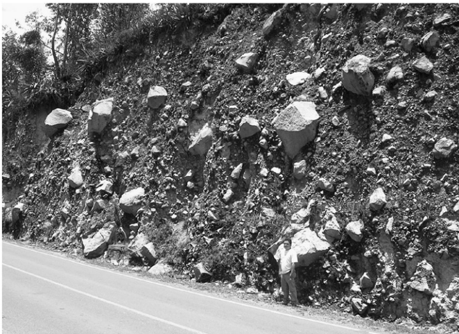
Fig. 6. Deposits of the Pre-Columbian rock avalanche exposed in a road-cut directly beneath the western edge of Cemetery Hill. Large angular boulders of granodiorite are set in a pulverized matrix. Note person for scale. The exposure is located in Fig. 5.
